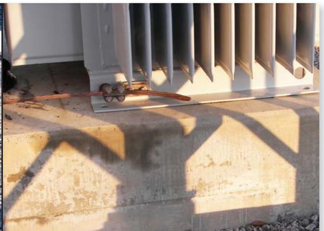
Thieves will steal coils of copper wire if they can get them; otherwise, they will go after the copper making up the grounds (left). Often, the criminals will just cut the sections off (right). The more enterprising thieves will tie the ground to a truck and see how much can be exposed before cutting.
